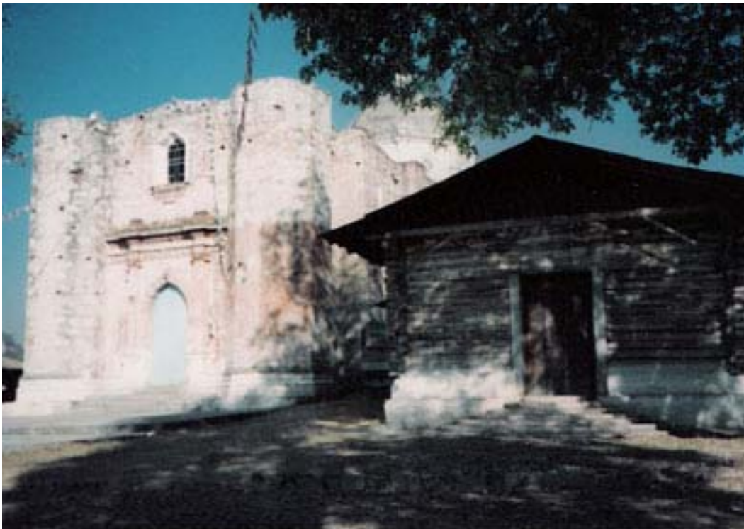
On the upper town of Tlaxiaco, a mix of 16 th century stone colonial architecture and the traditional log structures typical of the pre-colonial culture
