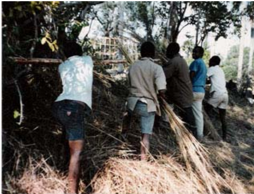
Gather elephant grass then strip the seed heads and most of the leaves after it's dried
