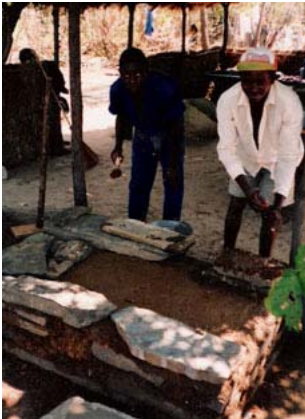
Building a stone and clay brick stove, my design
