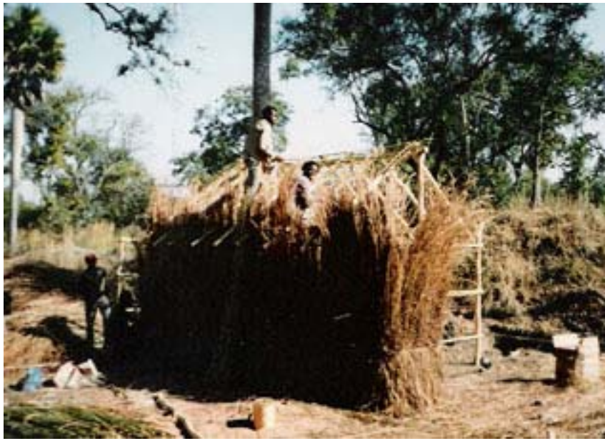
Tie the cleaned grass to the frame with small vines that pass for rope
